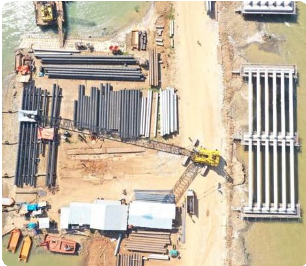
Title : Girder Installation
