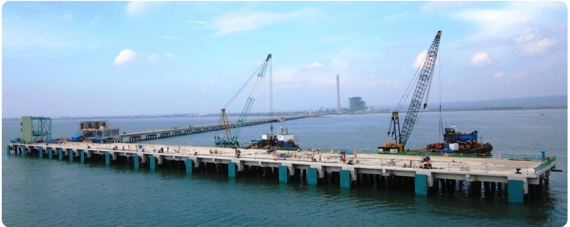
Title : Jetty 13,000 + Trestle 2km Year : July 2010
