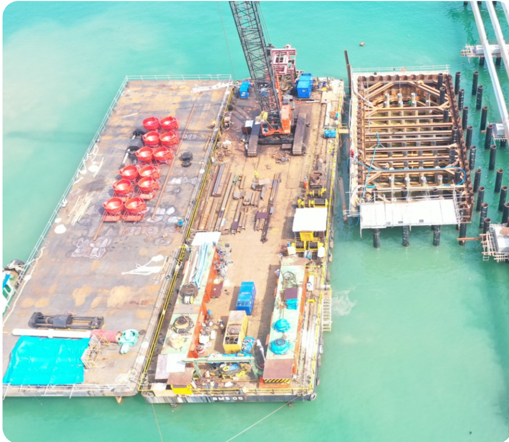
Title : Intake Pouring Concrete w/ Hopper
