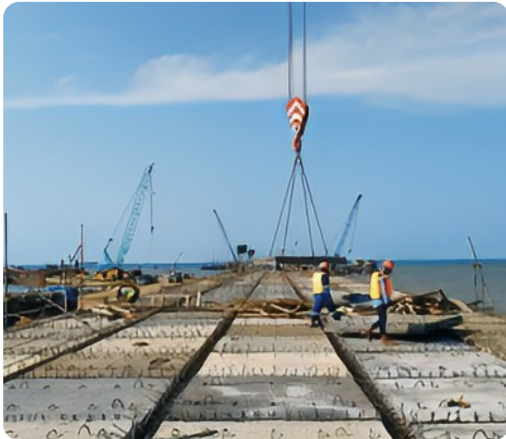
Title : Trestle Concrete
