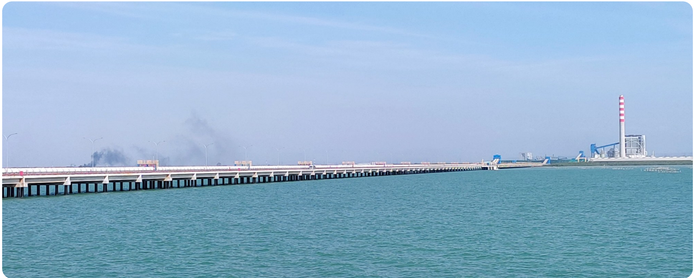
Title : Jetty 13,000 + Trestle 2km Year : July 2010
