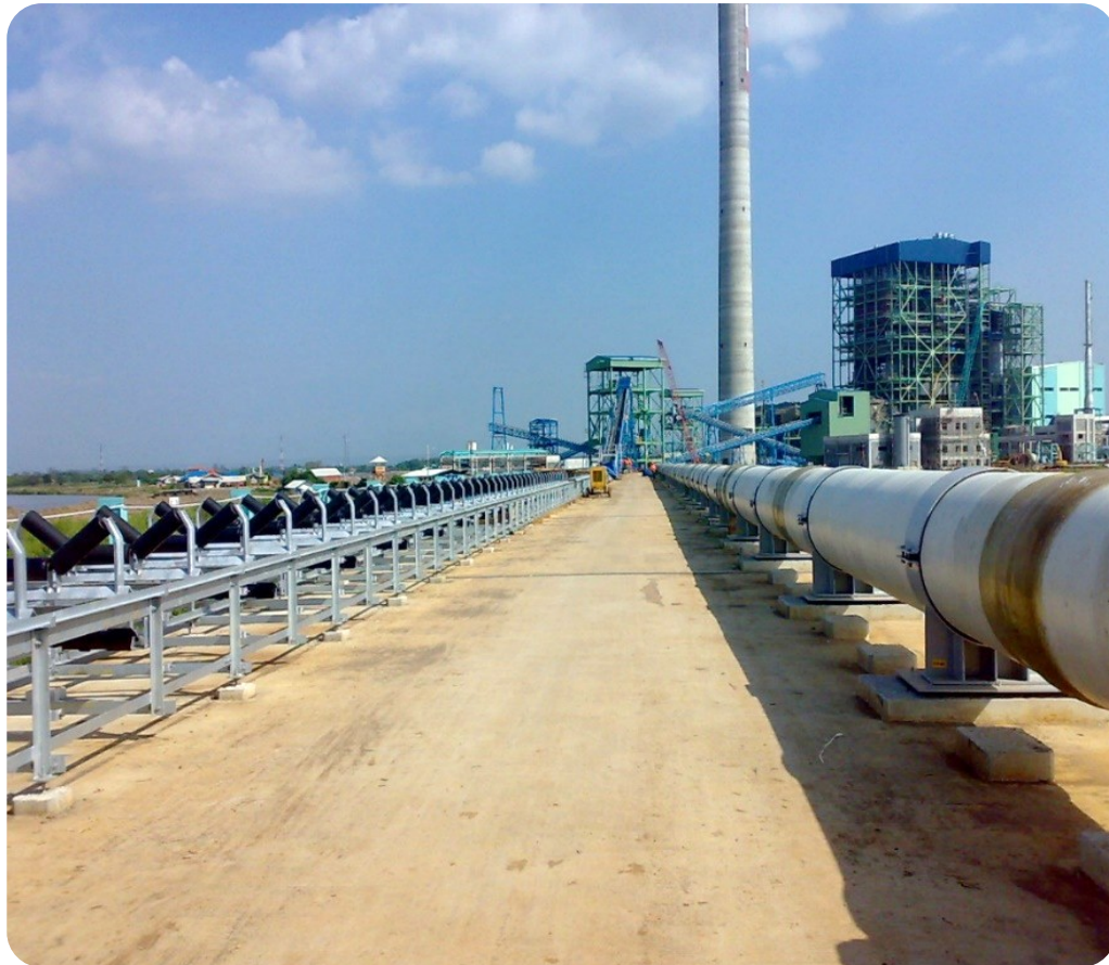
Title : Trestle + SWI Pipe
