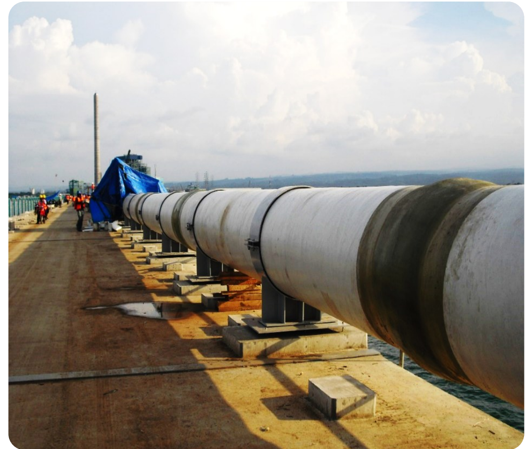
Title : Trestle + SWI Pipe
