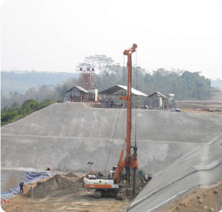
H-Beam Piling – September 2015
