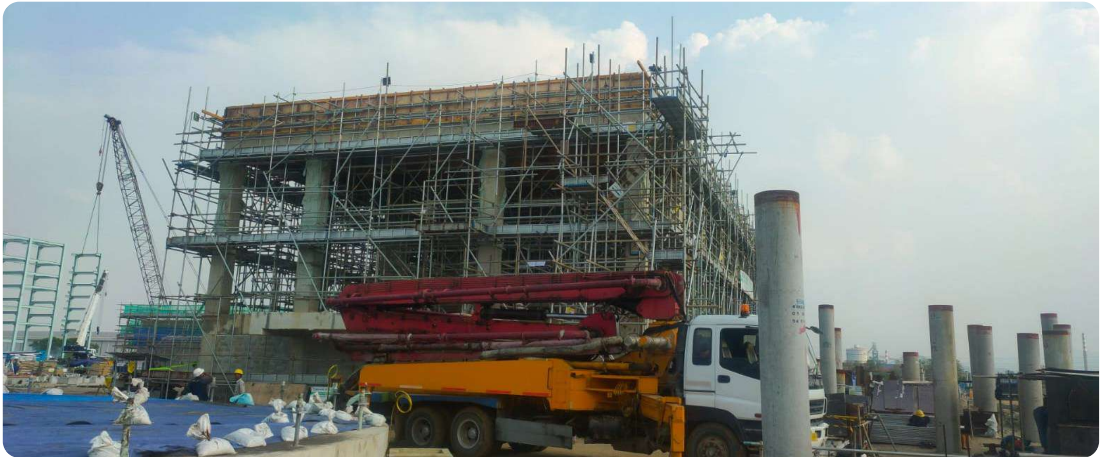
Pouring Concrete Parapet, Cable Trench Transformers, Sump Pit & Air Foundation – March 2023
