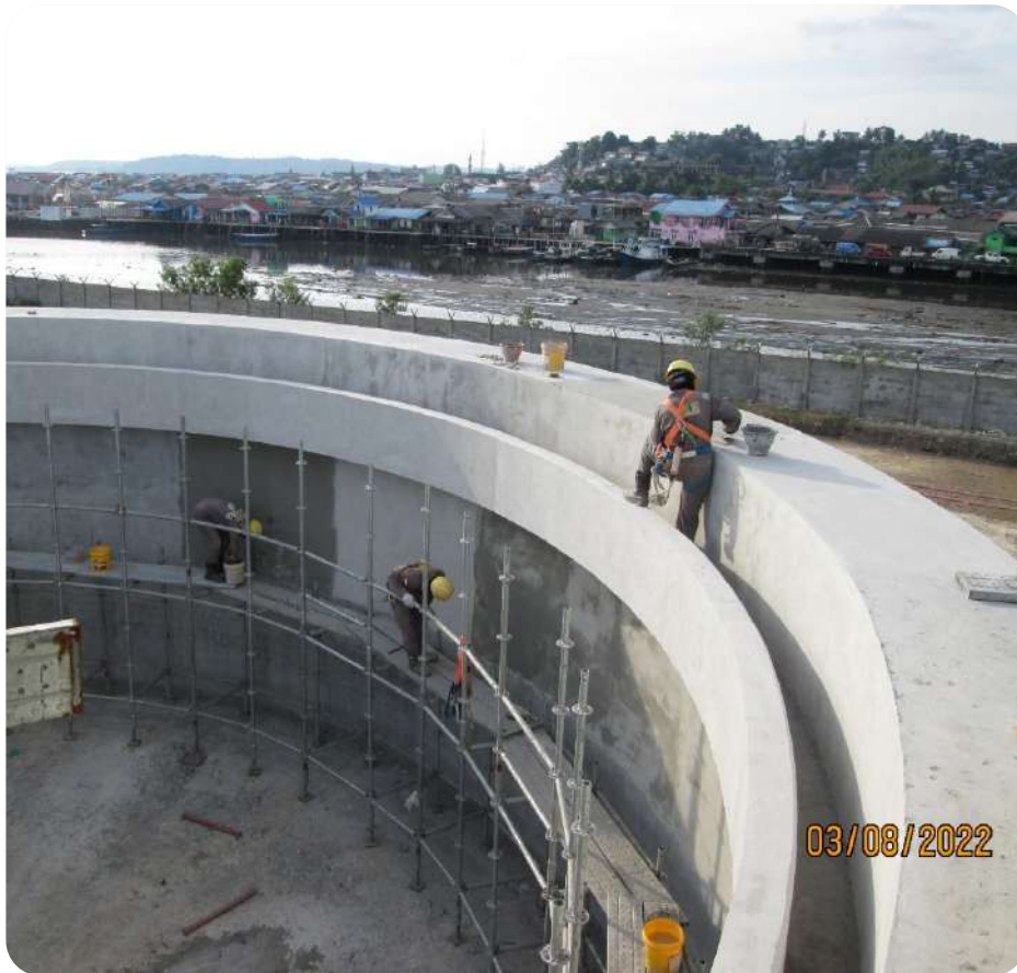
Clarifier Sludge Thickener – August 2022
