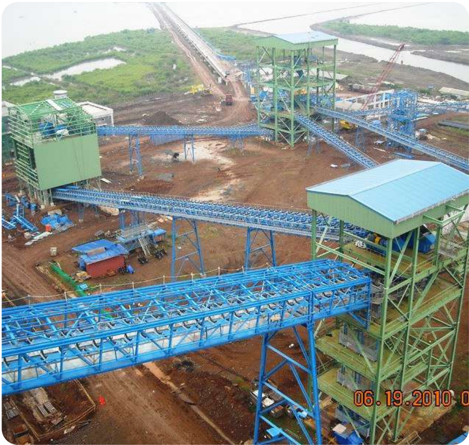
Belt Conveyor Erection – Year 2010
