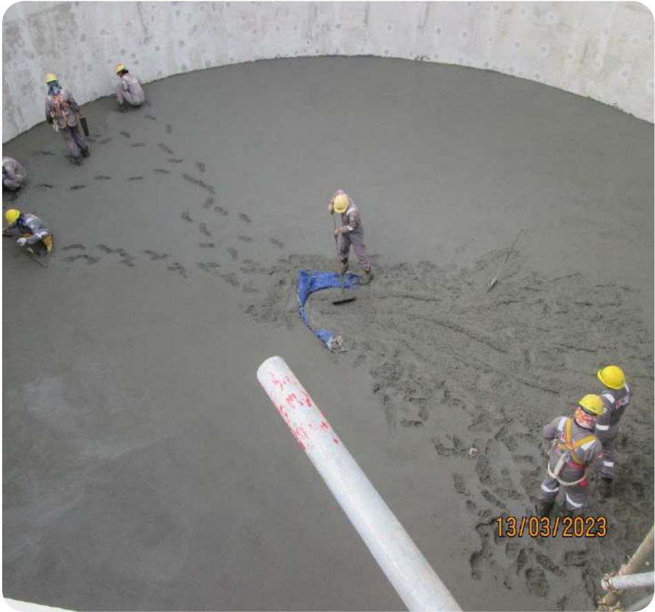
Concrete Slope Screeding — March 2023
